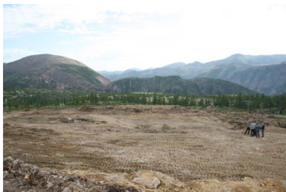
Process plant site preparation is well under way
