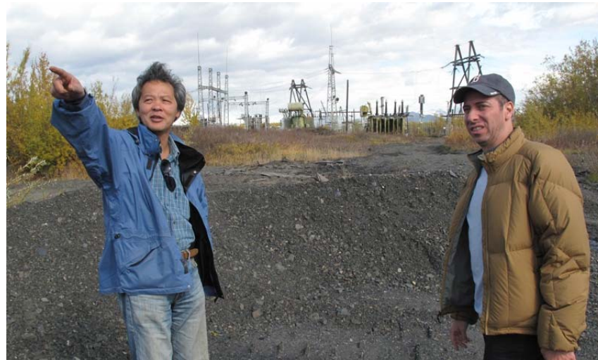
Ovoca team on license area, power transformer station in background
